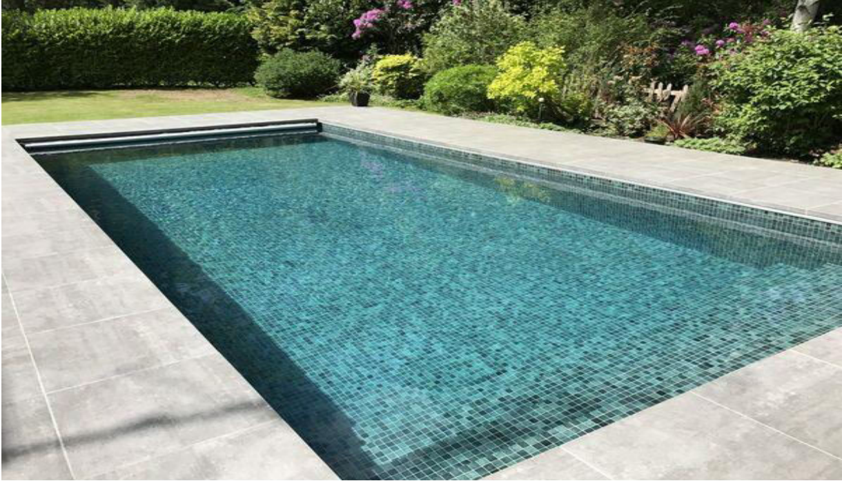
The walls of the pool will be faced with small mosaic ceramic tiles and there will be a limestone paving surround (see details below).
