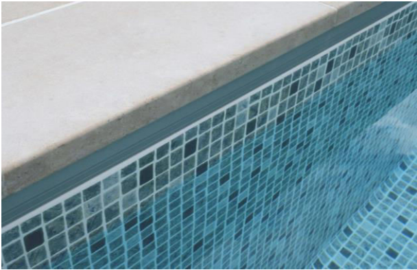
A mosaic of small grey and blue ceramic tiles will be used to face the walls of the pool, as above.
