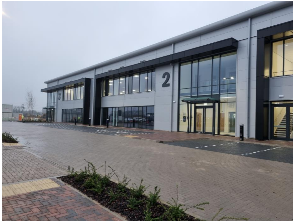
Trimotherm composite panel cladding, curtain walling, feature canopy & block paving
