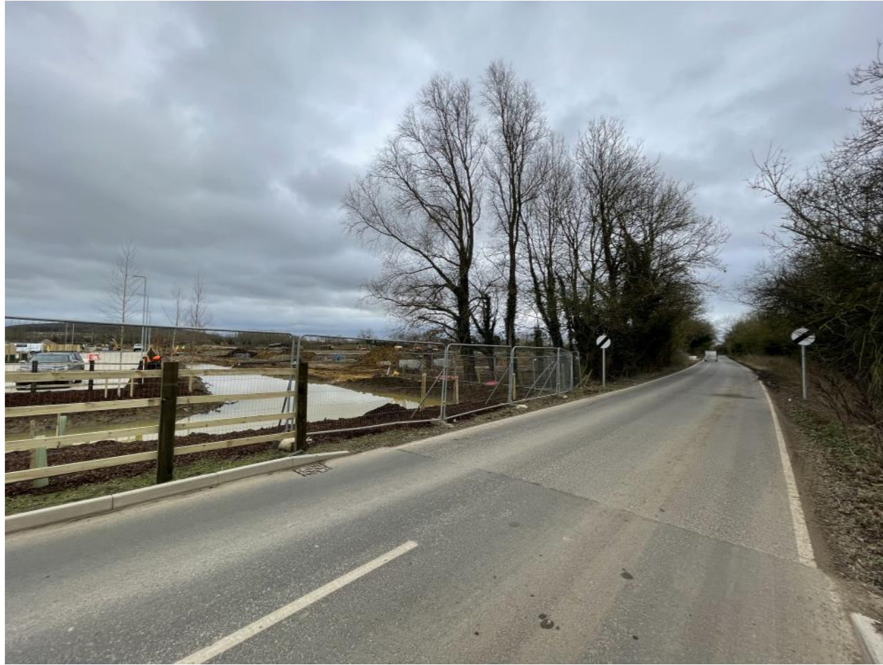
Fig. 07 Looking South along Wendlebury Road site frontage
