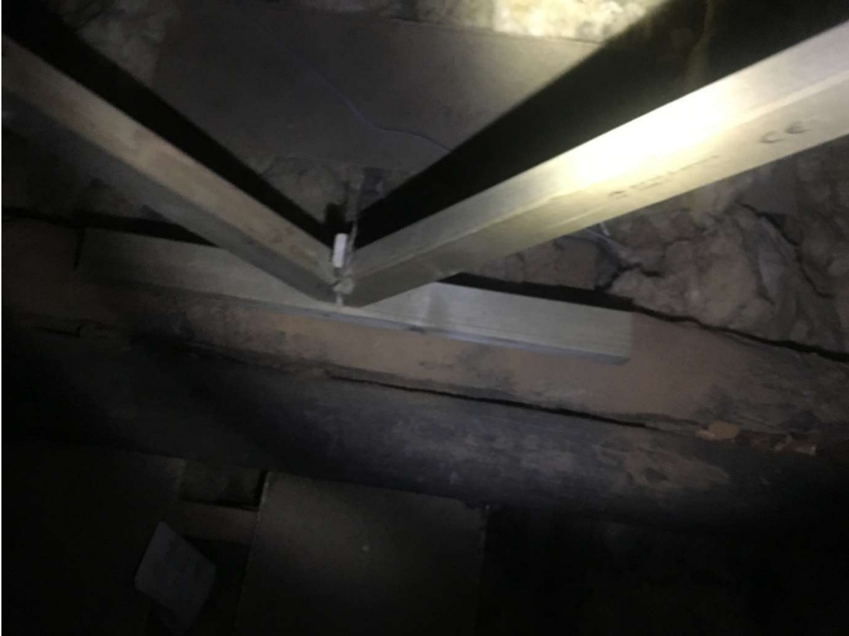
Photograph 7 - Truss 2 with modern bracing repair
