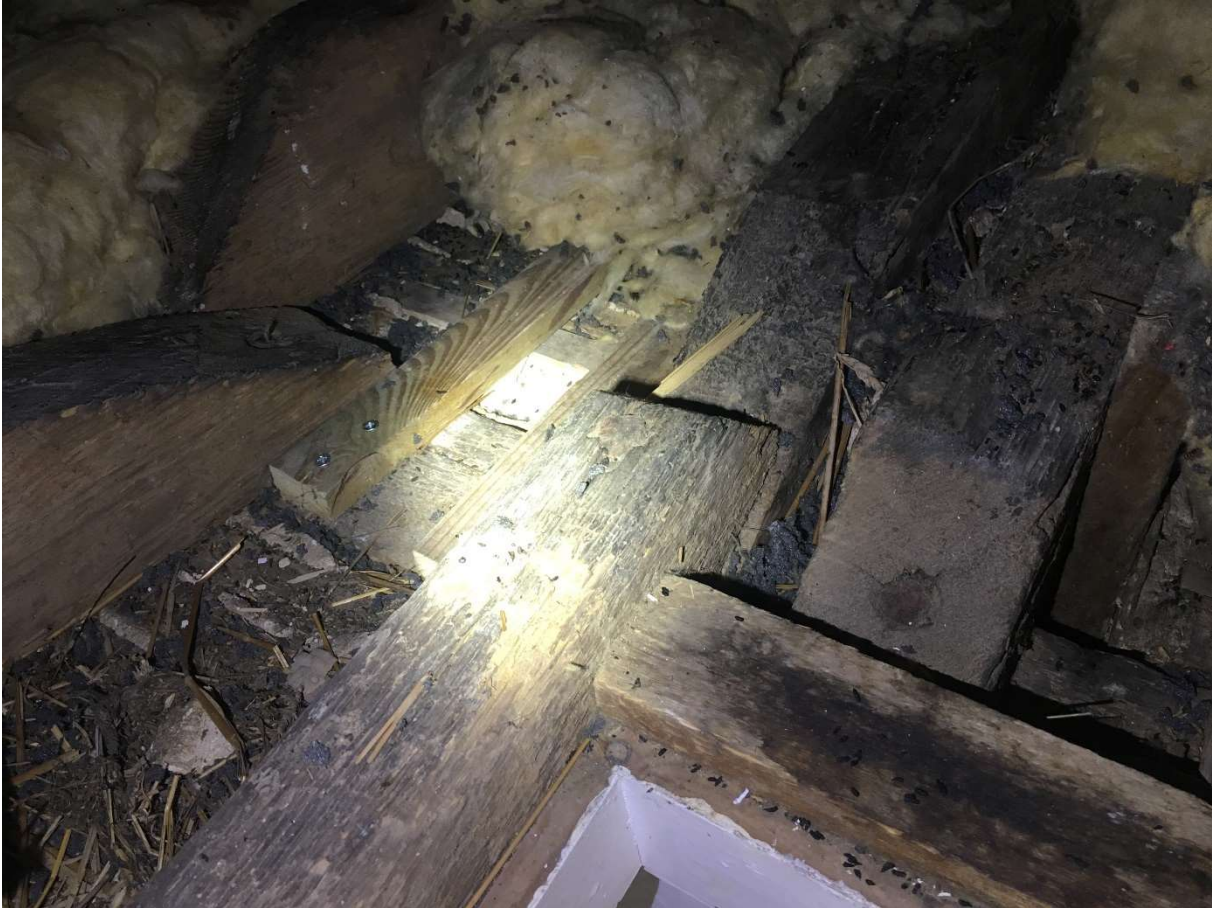
Photograph 9 - 4" x 3" attic floor joists bear onto walls below
