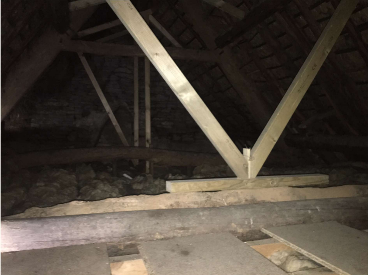
Photograph 3 - Truss 2 with modern bracing repair
