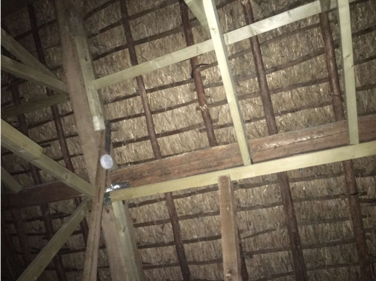
Photograph 2 - Modern C24 purlins an props support fir pole rafters
