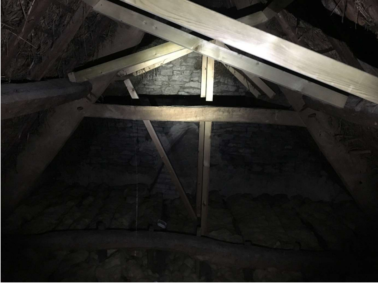
Photograph 6 - Modern C24 props
