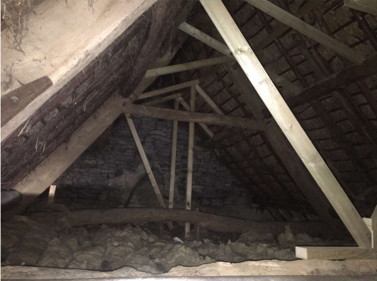
Photograph 1 - Original collar tie trusses and modern C24 strengthening props and purlins
