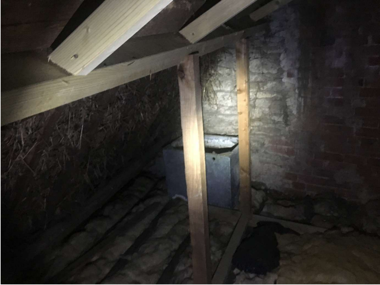
Photograph 8 - Modern vertical C24 props and purlin
