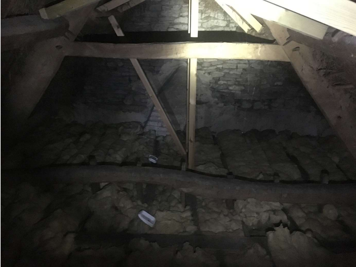
Photograph 5 - Truss 1 with modern C24 props beyond
