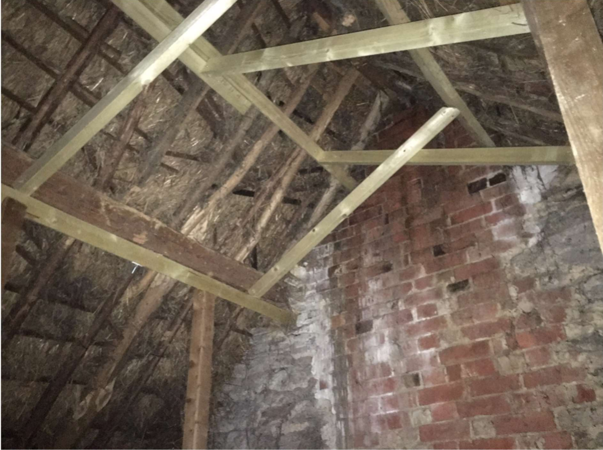
Photograph 4 - Modern C24 purlins and props
