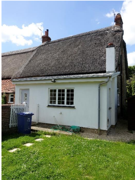
Fig. 2: Modern rear extension to No.1 Canal Yard
