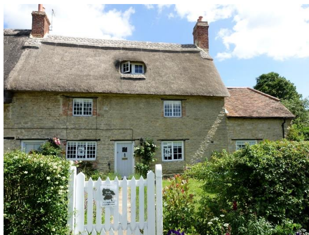
Fig.6: Existing dormer window to front elevation of No.3 Canal Yard – new dormer window to rear elevation of No. 1 to match
