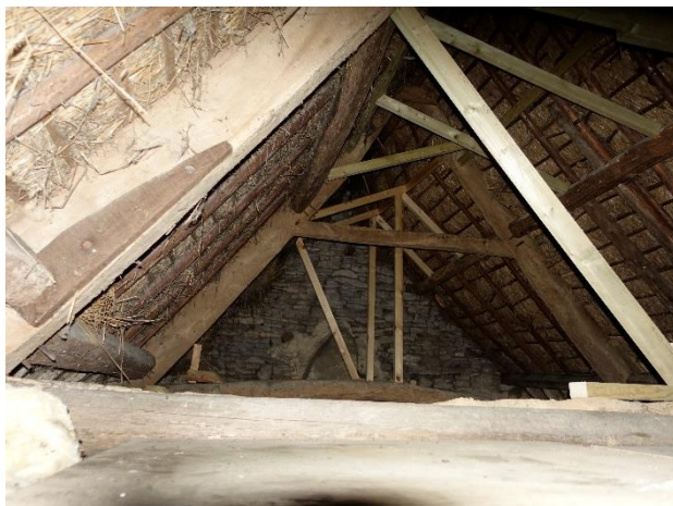
Fig. 4: Existing roof space over No.1 Canal Yard (Bedroom 3)
