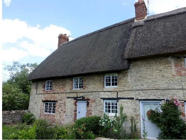
Fig. 1: Front elevation of No.1 Canal Yard (with adjoining No.2 Canal Yard)
