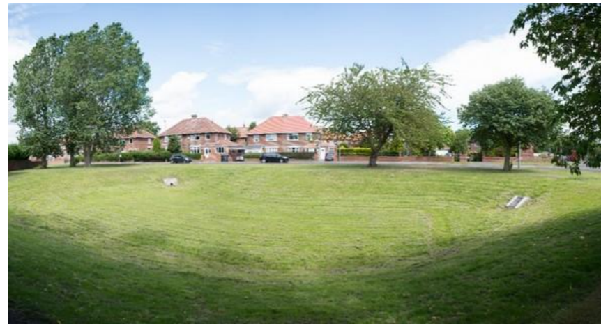
Figure 15: Example Image of Detention Basin
