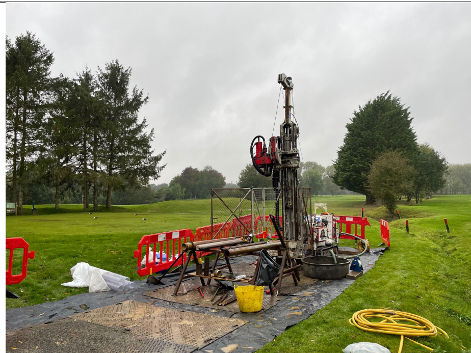
Photo 1. Photo showing typical rotary borehole rig setup
