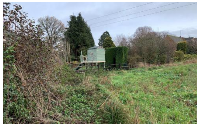
North east corner boundary partially open
