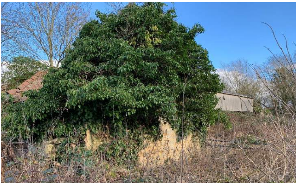
Remaining gable wall of Block G
