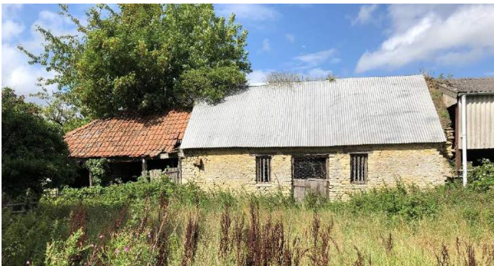
Blocks B and B1 on the opposite end of the farmyard
