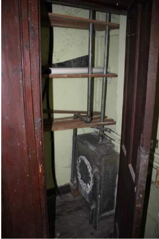
Plate 66: Lead tank in bathroom in F7 (left) and register in chimneybreast (right)
