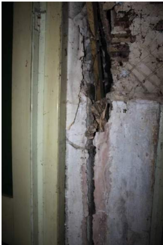
Plate 47: Vertical crack between rear wing (left) and outshut (right)
