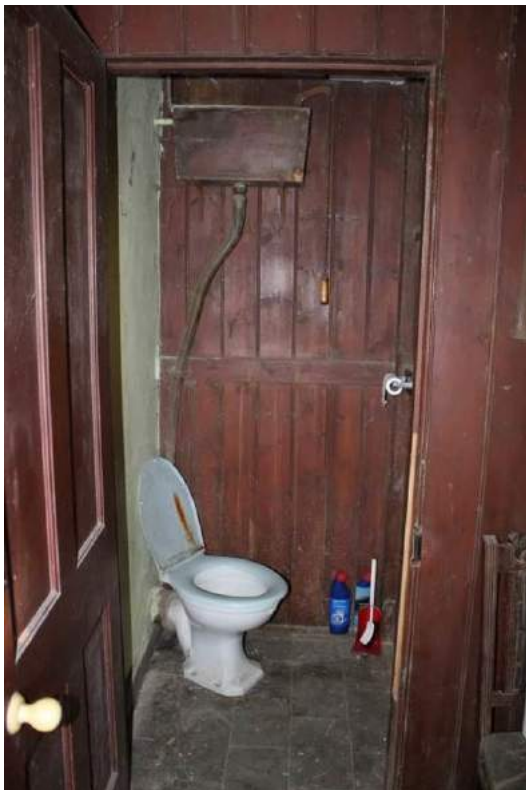
Plate 67: WC with wooden cistern in F7 (left) and partition between WC and bathroom (right)
