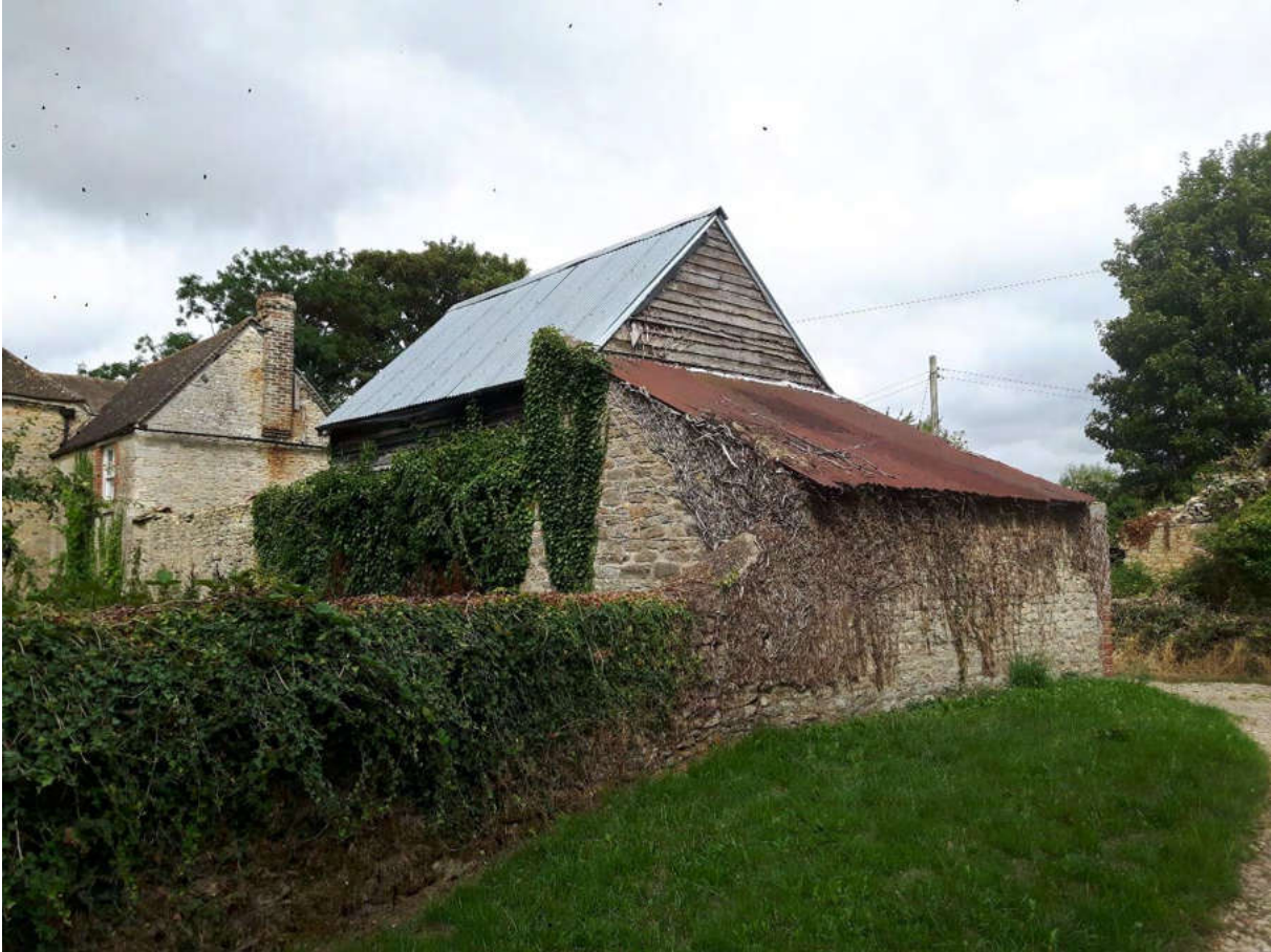
Photograph 19 - Block A, south-east elevation
