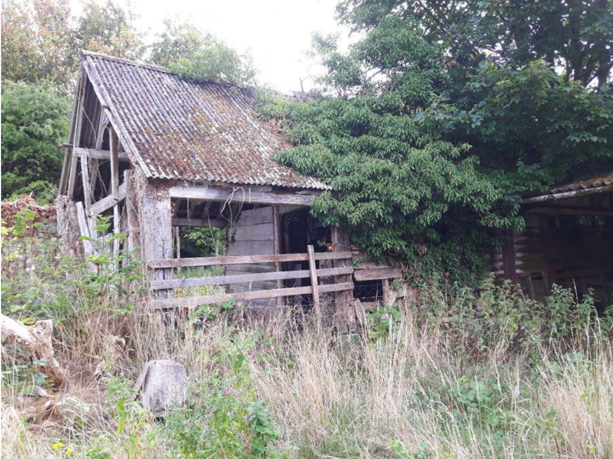
Photograph 31 - Block F, north west elevation
