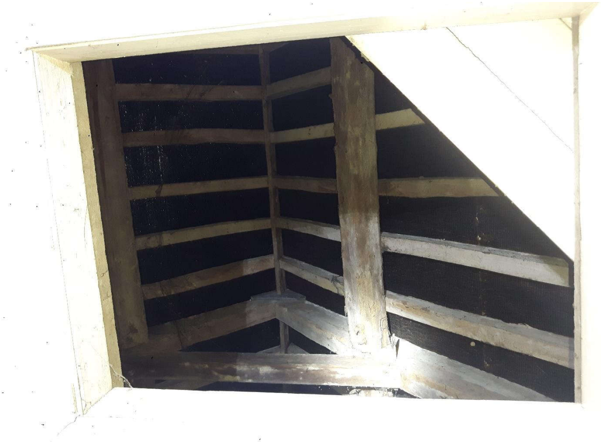
Photograph 15 - Roof structure showing primary rafters and ties forming A-frame
