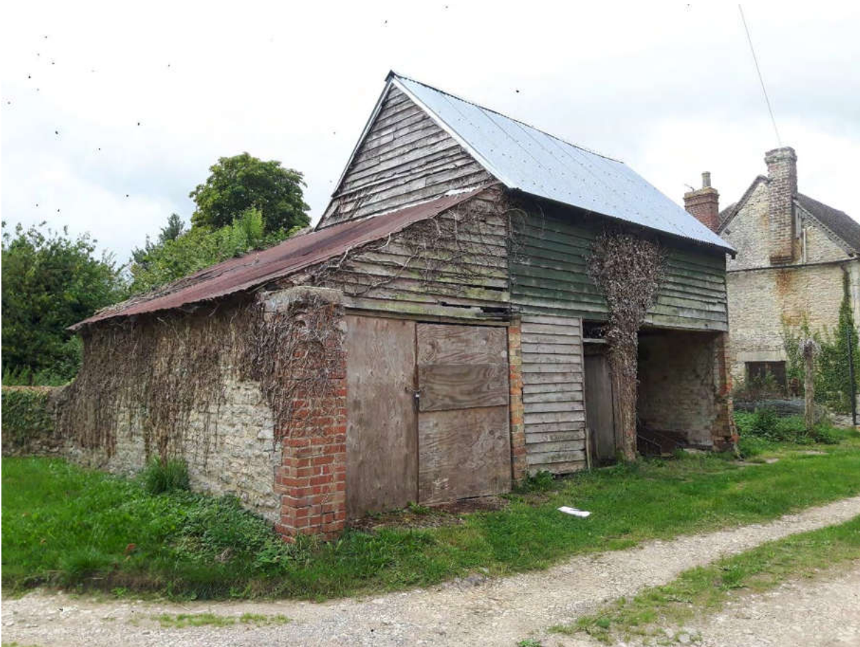
Photograph 17 - Block A, north elevation
