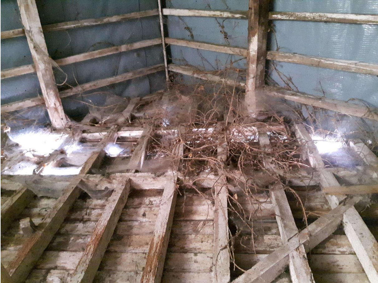
Photograph 21 - Block A, weather-boarded stud framing
