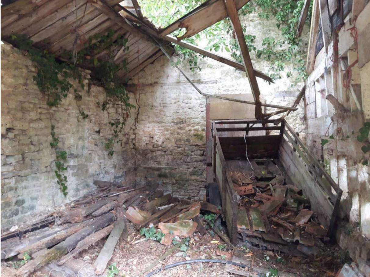
Photograph 26 - Block B1, internal
