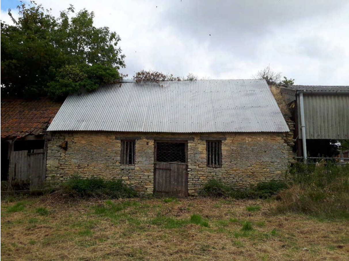
Photograph 21 - Block B, south elevation
