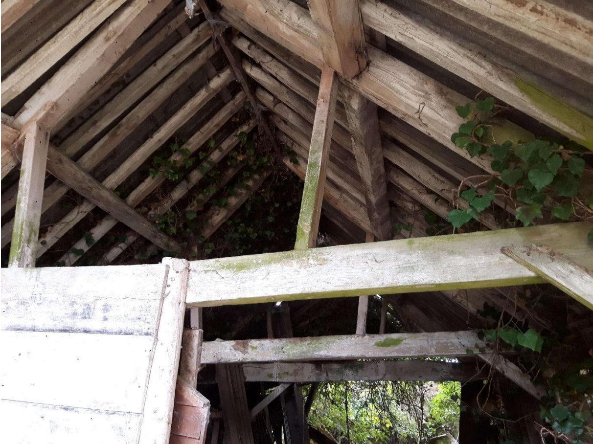
Photograph 34 - Block F, roof trusses looking south
