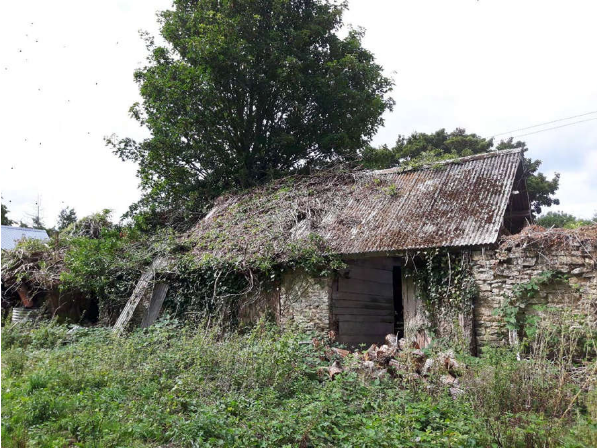
Photograph 32 - Block F, south west elevation
