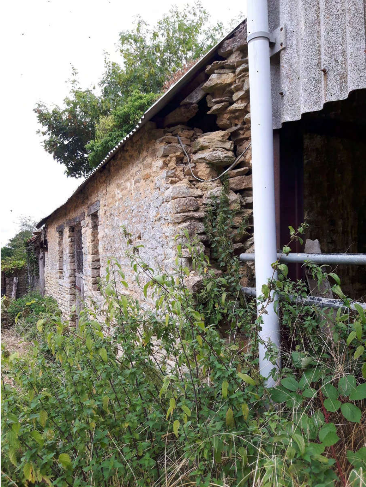
Photograph 22 - Block B, corner wall
