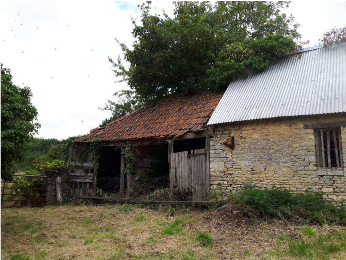
Photograph 25 - Block B1 , south elevation
