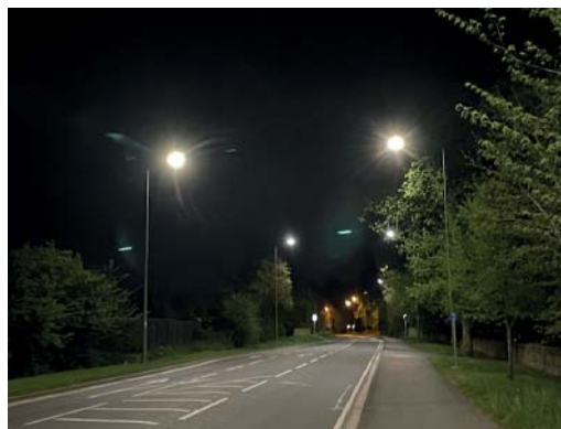
OXFORD ROAD (A44) - NIGHT LED street light, 4000K (~12m) Illuminance : 10-16 lux
