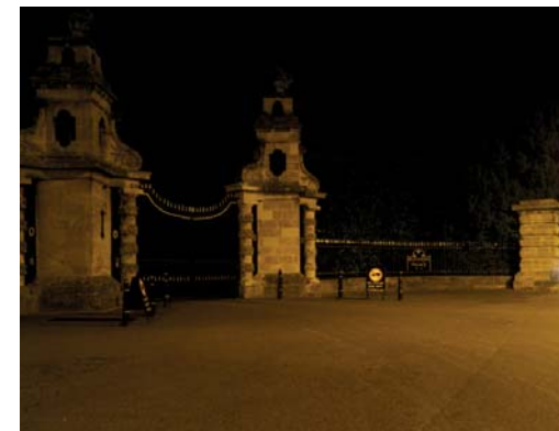
BLENHEIM PALACE ENTRANCE - NIGHT Light levels from street lights on opposite side of the road -Illuminance: 6 lux
