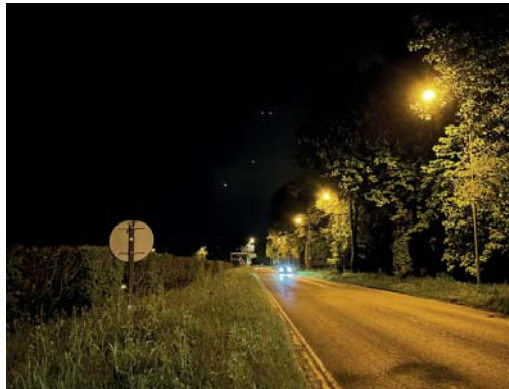
OXFORD ROAD (A44) ADJACENT TO SITE High pressure sodium street light (~12m) Illuminance: 4-26 lux
