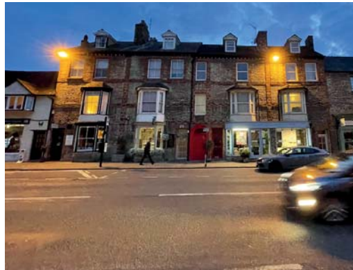
OXFORD STREET (A44) - NIGHT Wall-mounted high pressure sodium floodlights (at~9m) - Illuminance: 65 lux
