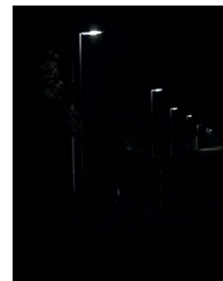
DIMMABLE LED STREET LIGHTS ALLOW ILLUMINANCE LEVELS TO BE REDUCED LATER IN THE EVENING.
