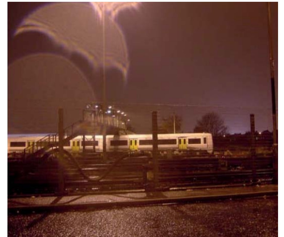
ILLUSTRATION: LIGHT SPILL FROM HIGH MAST LUMINAIRES
