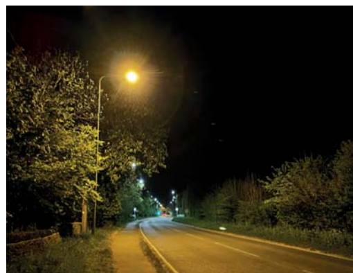
OXFORD ROAD (A44) ADJACENT TO SITE - NIGHT High pressure sodium street light (~12m) Illuminance: 4-26 lux
