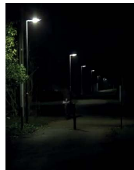
DIMMABLE LED STREET LIGHTS PROVIDE HIGHER LEVELS OF ILLUMINANCE WHEN TRAFFIC FLOW IS GREATER.
