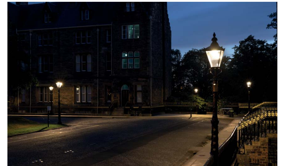
LIGHTING COLUMNS INSTALLED ON ONE SIDE OF THE SECONDARY ROUTES.
