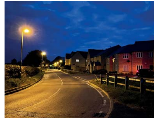
OXFORD ROAD (A44) - NIGHT High pressure sodium street light (~12m) Illuminance: 2-16 lux
