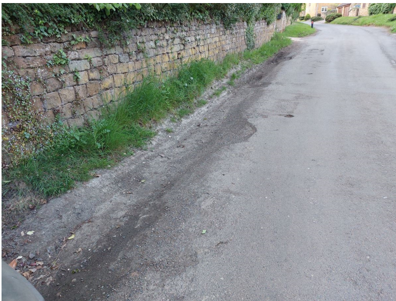
Image showing damage to the grass verge on Wroxton Lane caused by parked cars
