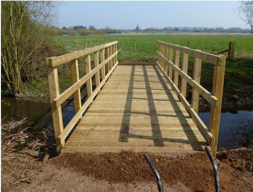
Previous timber footbridge installation as a typical example
