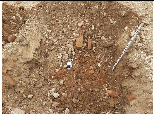
25.04.22 – S3 Soil Excavation
