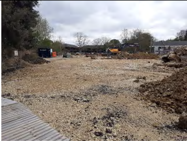
25.04.22 – Eastern view along the northern boundary
