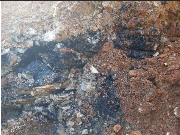
25.04.22 – Black stained soils around broken out slab
