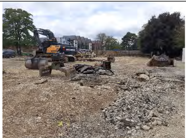
25.04.22 – Breaking out of relict drainage at a central location near the southern boundary
