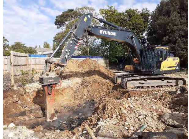
25.04.22 – Breaking out of slab at base of interceptor
