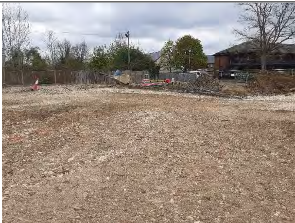
25.04.22 – View to the northwest corner where remedial works of HS1 completed
