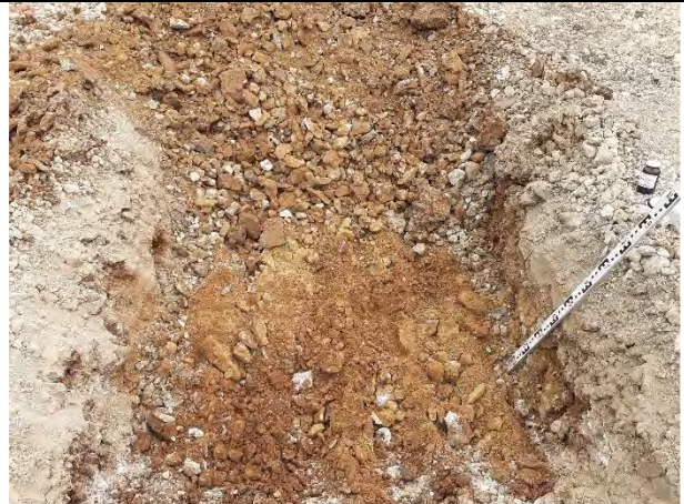
25.04.22 – S4 Soil Excavation
