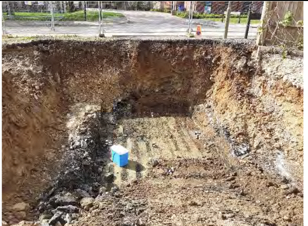
25.04.22 – Remediation excavation following removal of impacted soils
