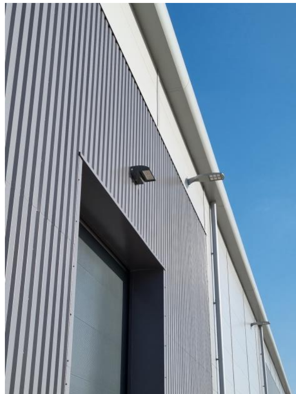
Vertical metal profile cladding & loading door
