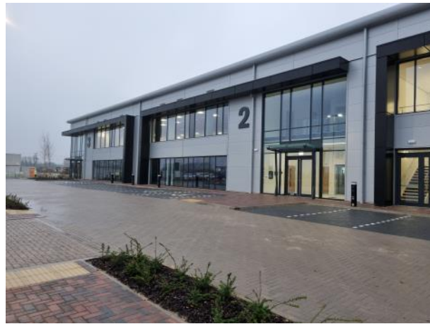
Trimotherm composite panel cladding, curtain walling & feature canopy
