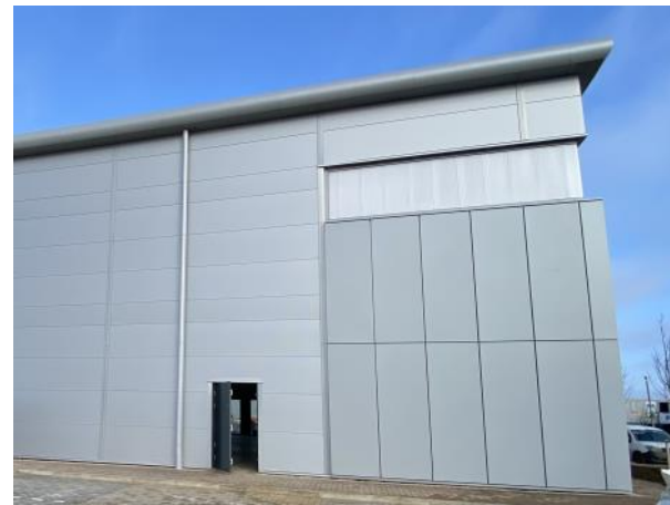
PPC aluminum rainscreen & translucent cladding
