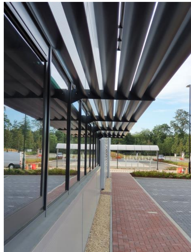
PPC aluminium glazing & brise soleil
