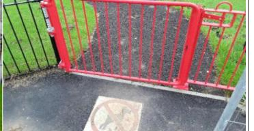
Finding: The gate is closing too quickly (less than 4 seconds)
