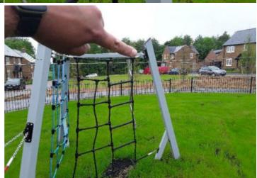
**Finding:** There is/are finger entrapment/s in the frame due to missing inserts and the item fails to meet the requirements of BS EN 1176 Part 1 4.2.7.6 Entrapment of fingers
