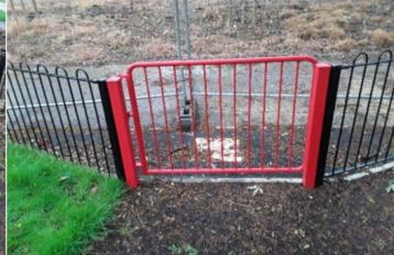
Action: Take corrective action to ensure that the gate closes in 4-8 seconds
