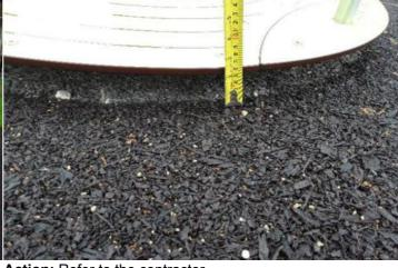
**Finding:** The distance between the underside of the roundabout platform and the playing surface is less than 60mm and contravenes the requirements of BS EN 1176 Part 5 which requires that the distance be maintained between 60mm-110mm for the entire circumference of the roundabout ( measurement between the surface and the underside of the roundabout platform is 50mm)
