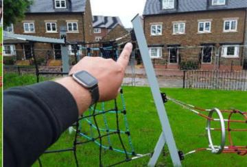
**Finding:** NOTE - There are fixings missing on a climbing net **Action:** Complete the installation (currently secured by cable ties)
