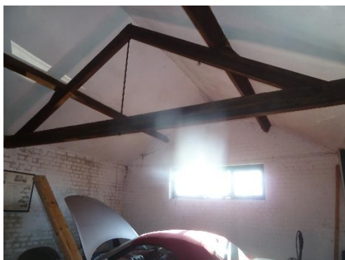
Photo 18: Building 5 interior - vaulted and plaster-boarded garage
