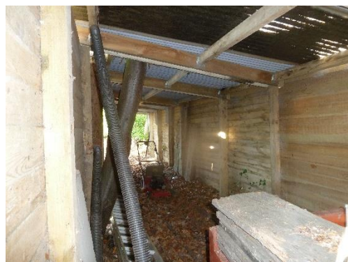
Photo 22: Interior of building 7, looking west
