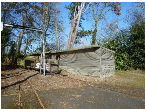
Photo 21: Building 7, southern elevation
