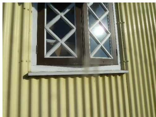
Photo 4: Open window providing access into interior of building 2
