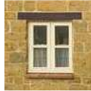
Timber window headers to most openings. Dressed stone cills.
