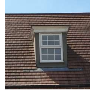
Flat roofed dormer with slim cheeks and a window of a smaller scale to the one below
