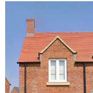
Pitched gablet with roof covering to match main roof
