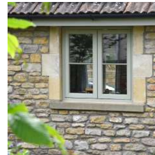
'Cottage' style flush fitting casement windows with a vertical emphasis
