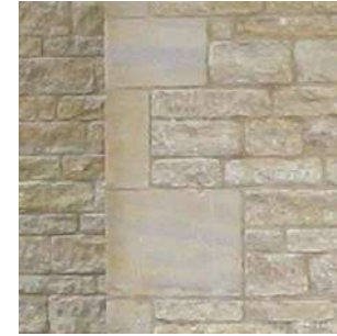
Dressed limestone quoins
