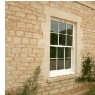
Dressed limestone window surround with Georgian style sash window
