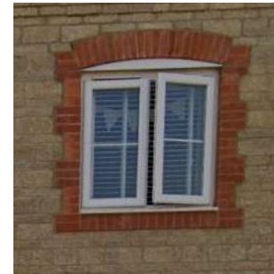
On key stone dwellings, red brick window surrounds with red brick cill would be fitting
