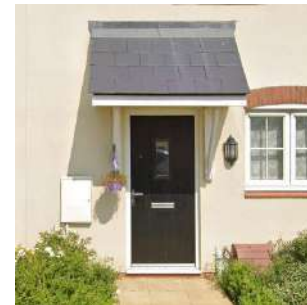
Appropriately proportioned porch canopies supported by timber brackets. Pitched, mono-pitched and flat would all be suitable
