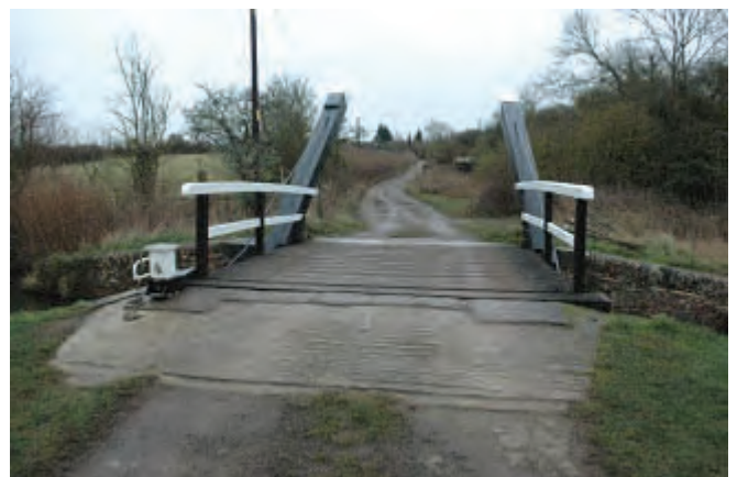
View from Bridge 231
