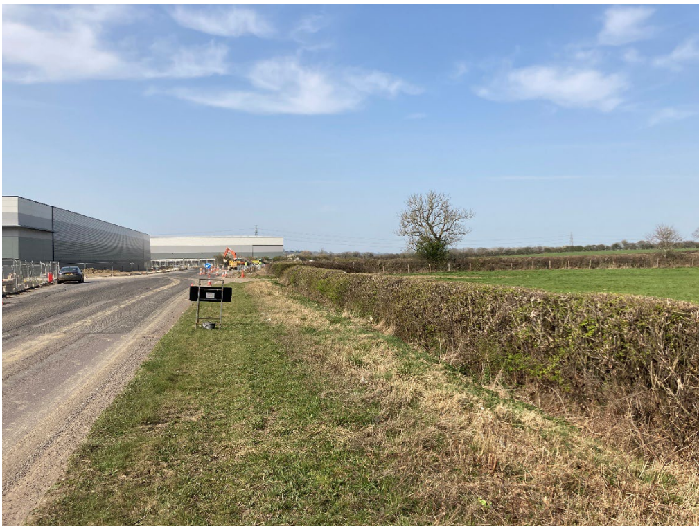
Photograph 8 - Looking north-west towards new development across A361
