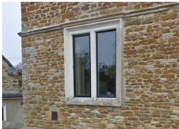
Metal window with carved limestone reveal
