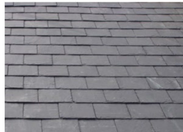
Welsh slate roof
