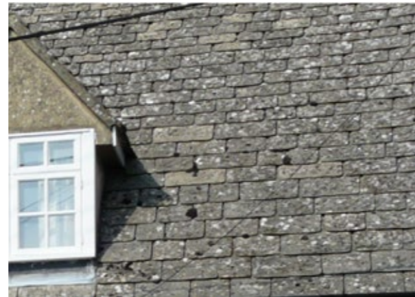
Stonefield slate roof
