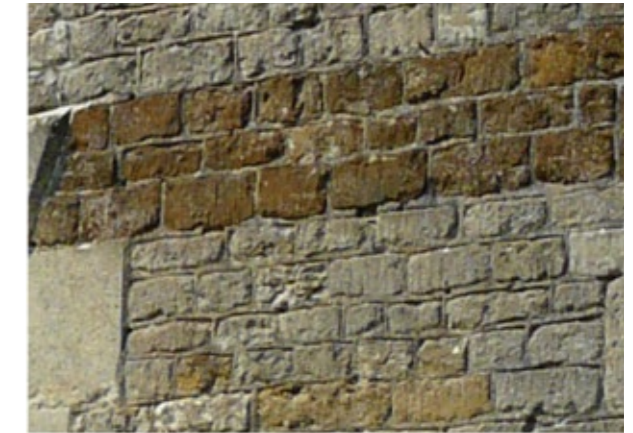
Limestone Blocks with Ironstone Banding
