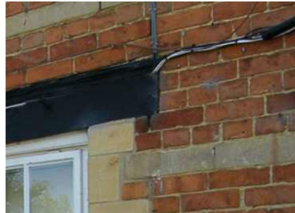
Brick with Limestone Ashlar Dressings
