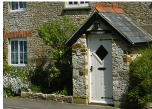
Timber panel door
