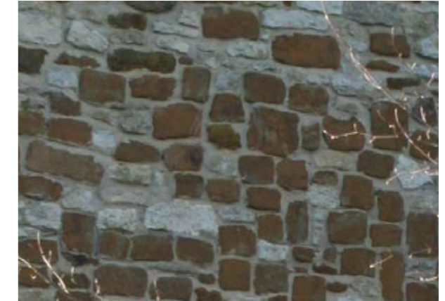
Random mix of ironstone and limestone blocks
