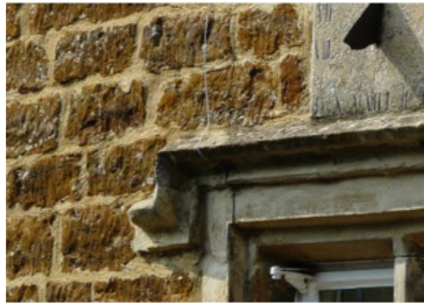
Ironstone Blocks with Limestone Lintel and stone mullions
