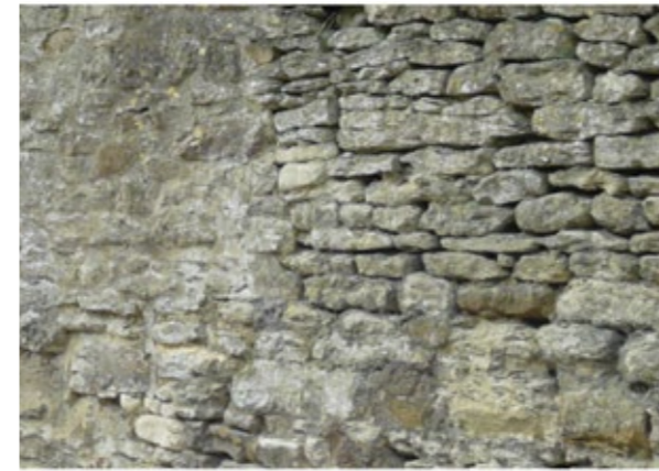
Rubble Limestone of a boundary wall
