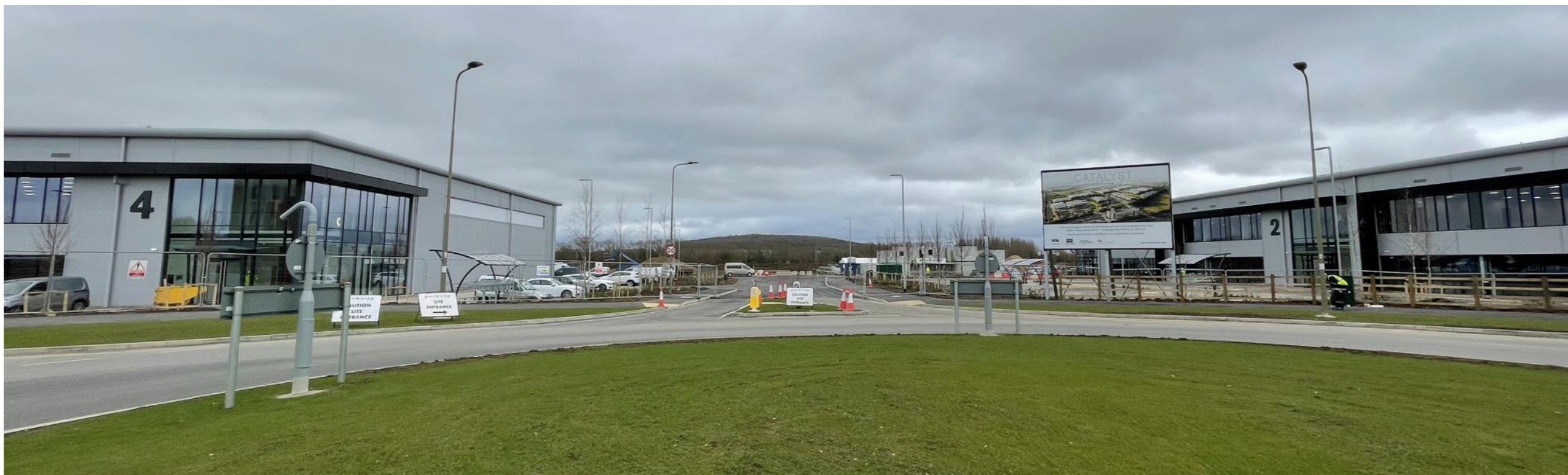
Fig. 02 Site entrance from the new roundabout on Wendlebury Road
