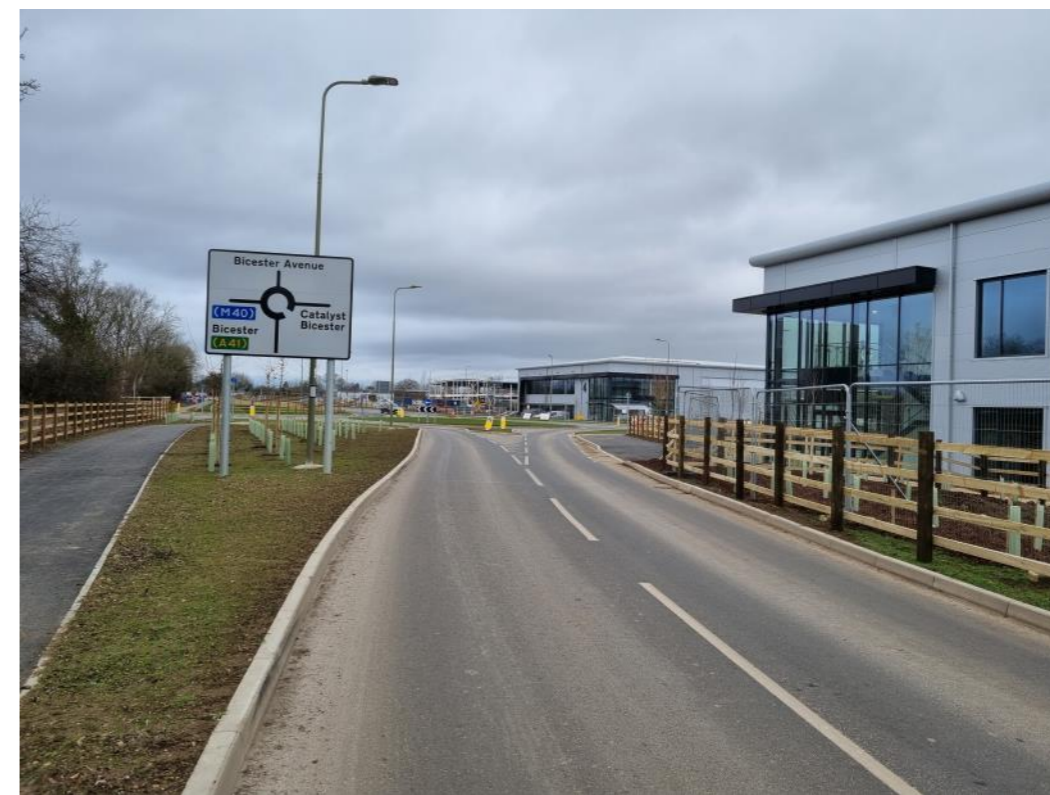
Fig. 04 Looking North along Wendlebury Road
