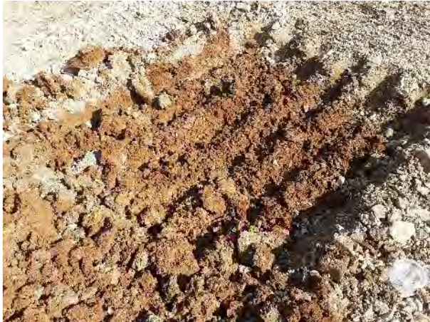
20.04.21 – Inspection of surface soils within ACM hotspot area. No visible ACM observed.
