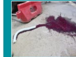
3 Contain the source of the spill and prevent spreading and entering drains
