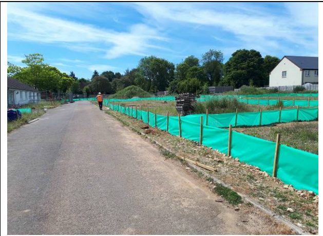
02.06.20 – Southern view down access road
