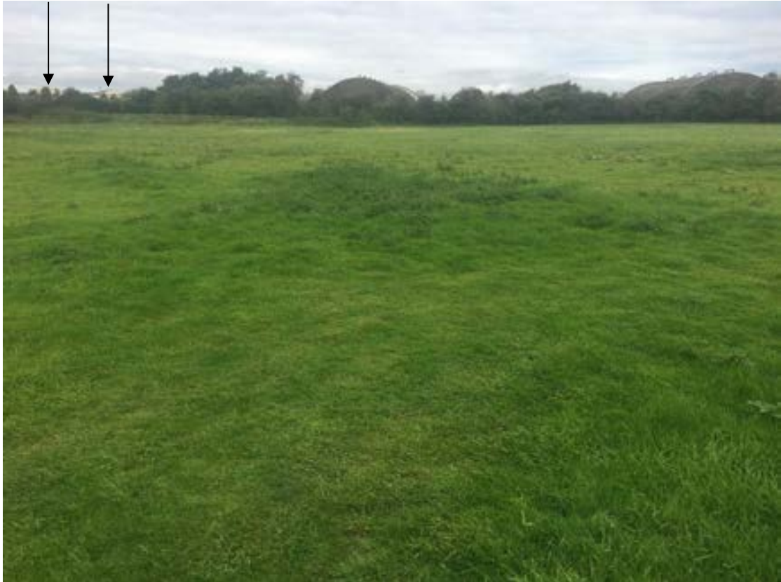
Plate 9: Looking north from the Site's northern field towards two Hardened Aircraft Shelters (centre) and partial views of an Aircraft Maintenance Hanger and Engine Test Shed on far LHS (black arrows).
