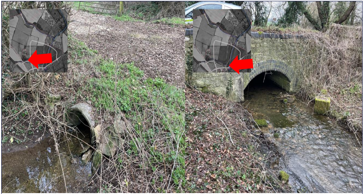
Figure 5-2: Hydraulic structures at West watercourse
