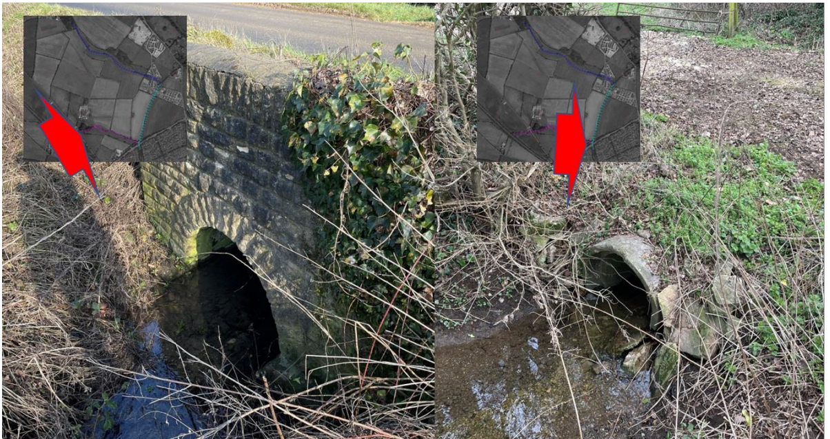
Figure 5-3: Hydraulic structures at West watercourse
