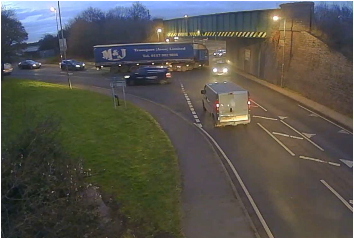
Figure 3.5 – Observed Articulated Vehicle Movement through Southern Junction
