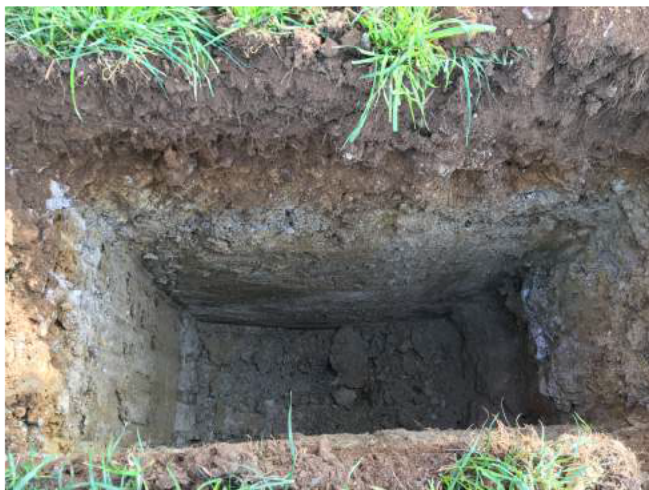
Photo 7: Excavation of trial pit IT04.
