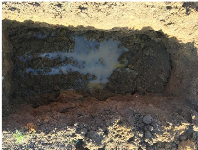
Photo 5: Excavation of trial pit IT03.
