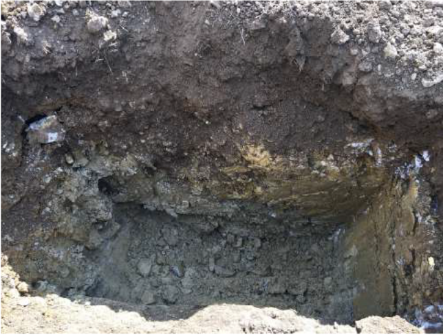
Photo 1: Excavation of trial pit IT01.
