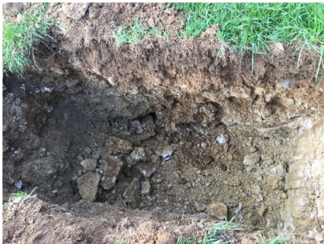
Photo 23: Excavation of trial pit IT12.
