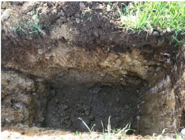
Photo 9: Excavation of trial pit IT05.
