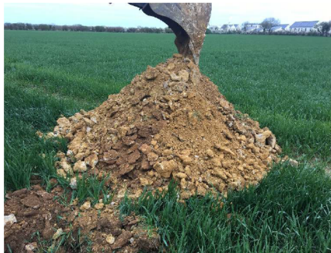
Photo 16: Arisings from trial pit IT08.
