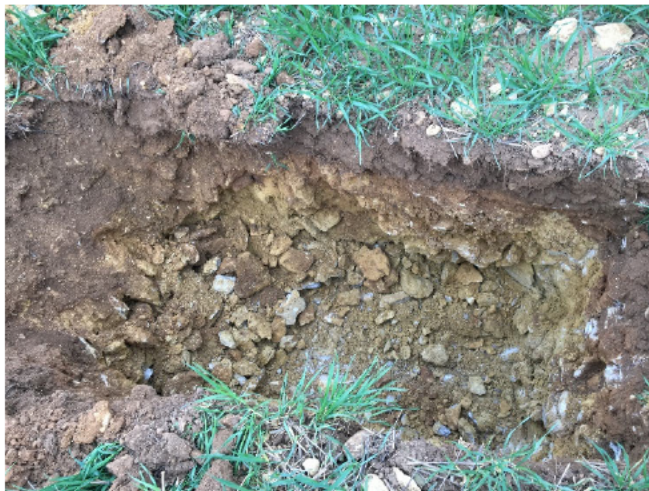
Photo 13: Excavation of trial pit IT07.
