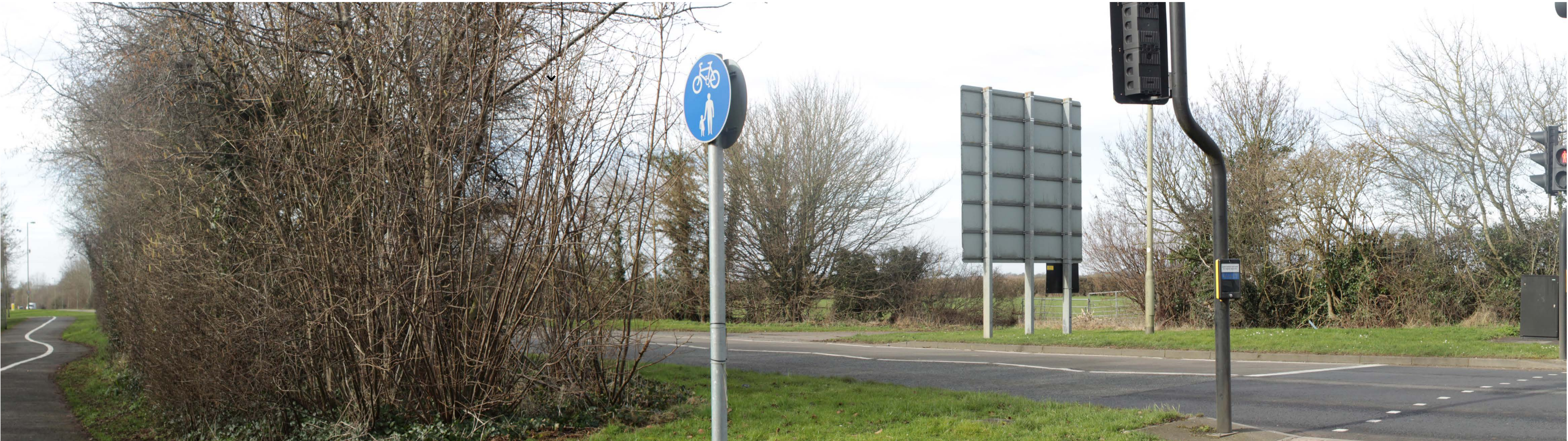
Photo Viewpoint 5c: View from A4095 near the A4095-B4100 roundabout
