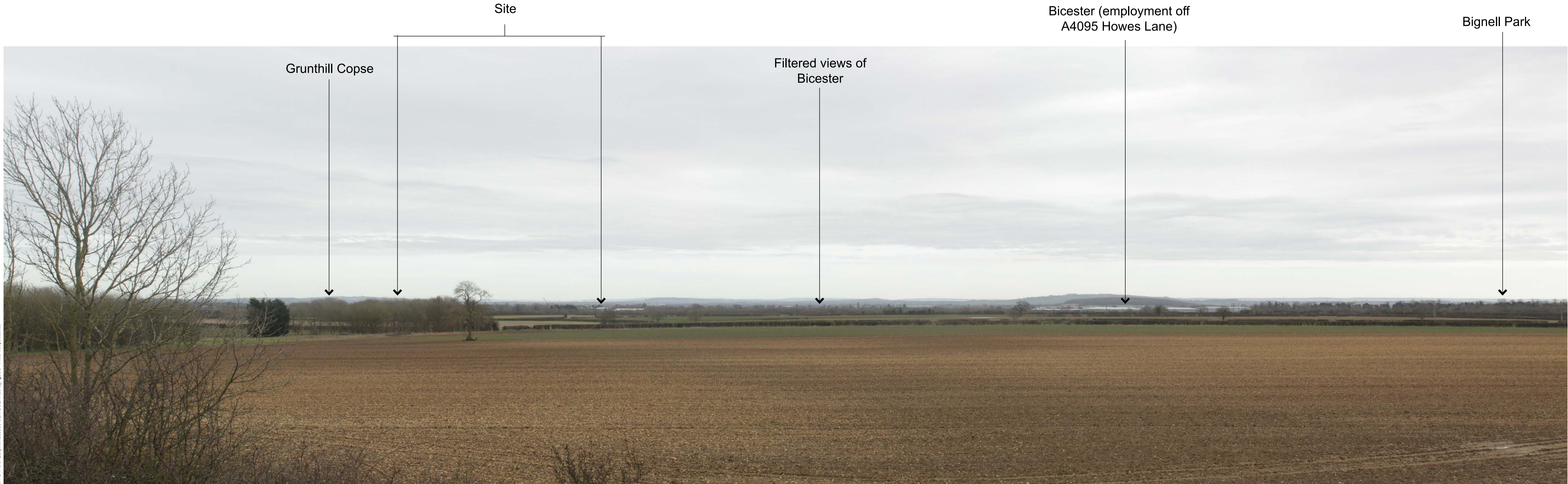
Photo Viewpoint 12: View from Middleton Road over M40 Motorway
