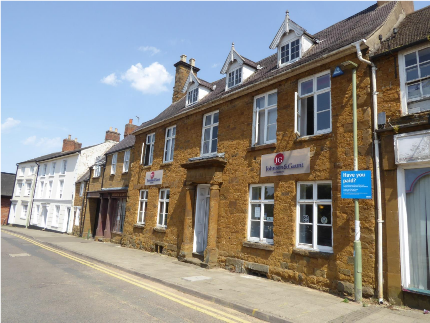
Figure 3 East side of North Bar Street, south of appeal site
