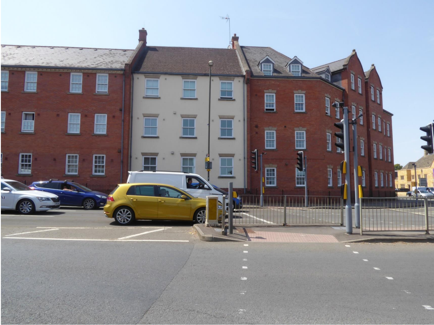
Figure 2 Block of apartments at Warwick Road junction
