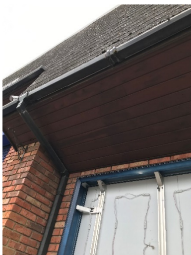
Photograph 3: Eastern aspect of building showing wooden soffits.
