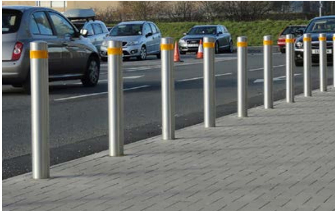
Bollards for pedestrian safety
