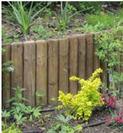
Sustainable material retaining wall
