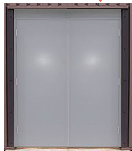
01: New fire escape doors
