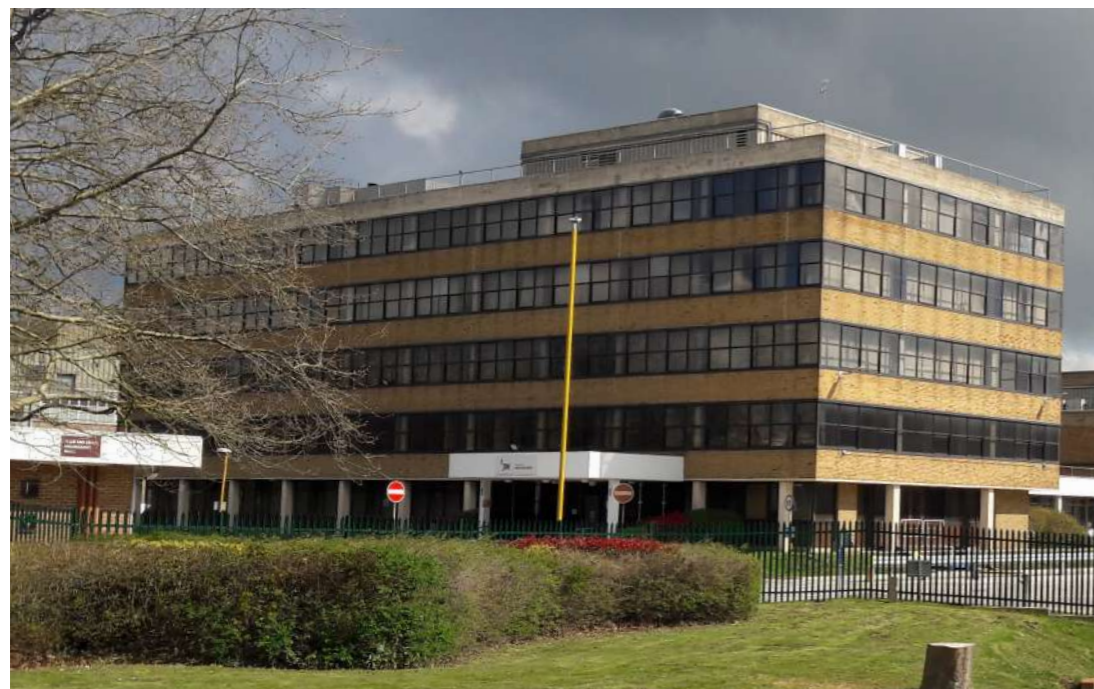
01: Demolition of the existing Main Office Block
