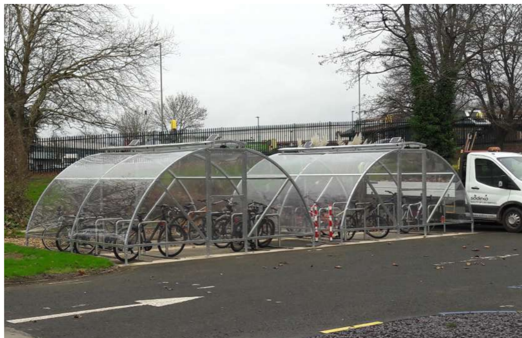
Relocated 2nr. bicycle storage shelters
