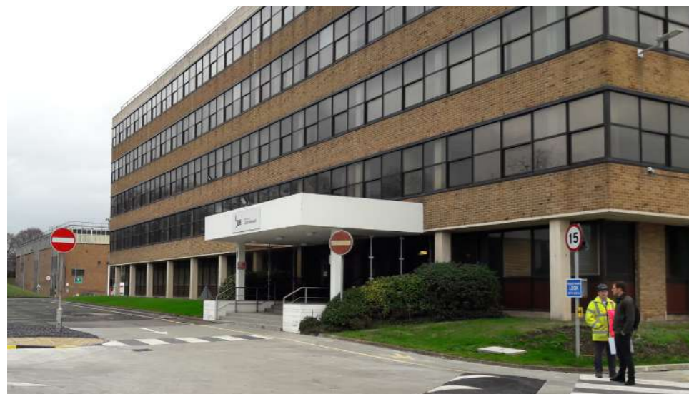
05: Main Office Block - View from site main entrance
