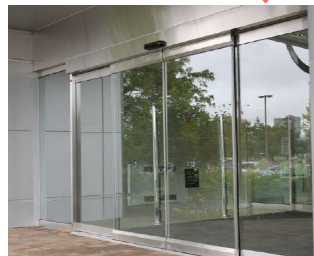
03: New double sliding entrance door
