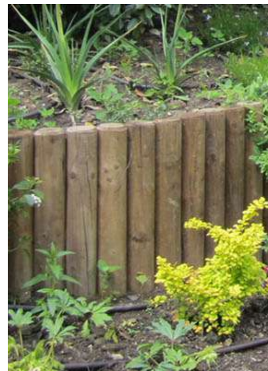
Sustainable material retaining wall
