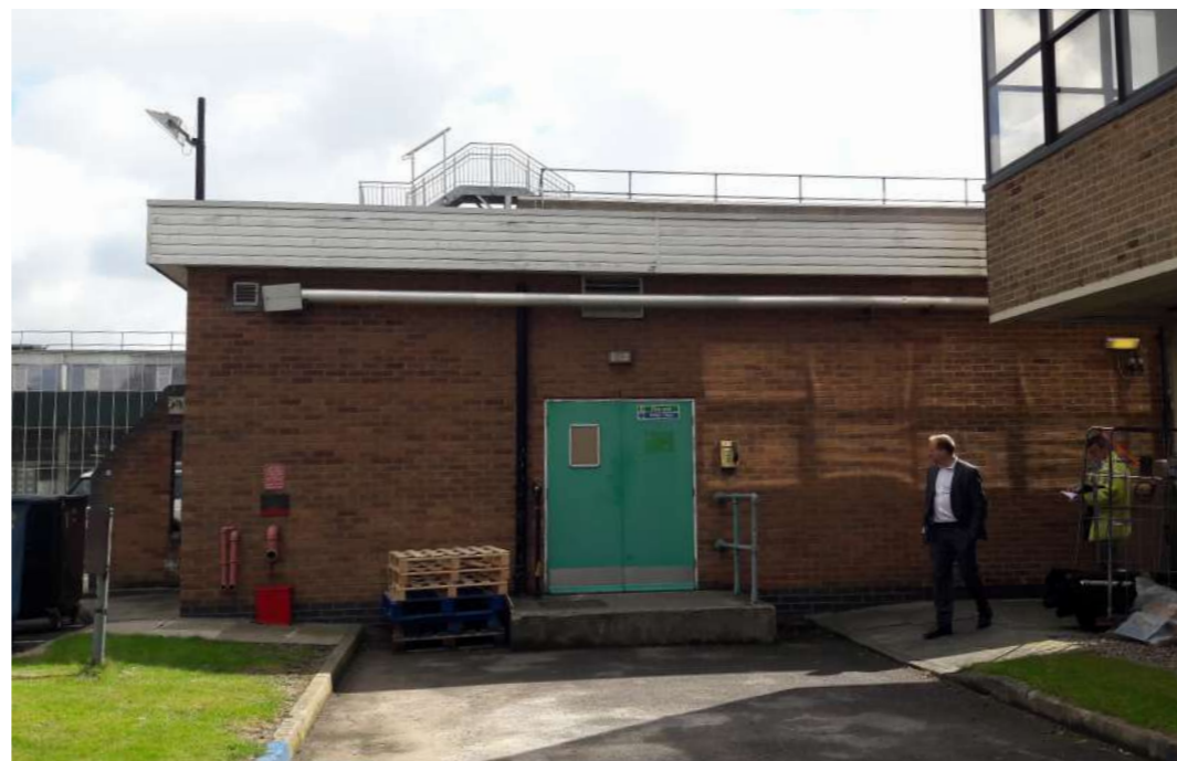
02: Recladding of Computer Suite facade
