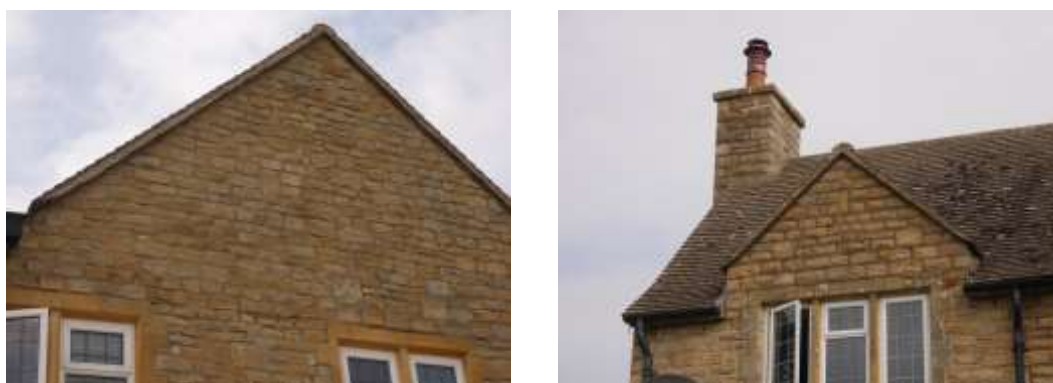
Figs. 9 & 10 Verge and chimney base fully pointed
