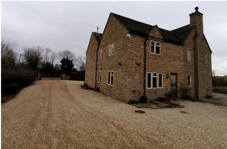
North & West Elevations. Entrance gates seen in background.
