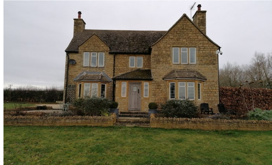
South Elevation - Original House.
