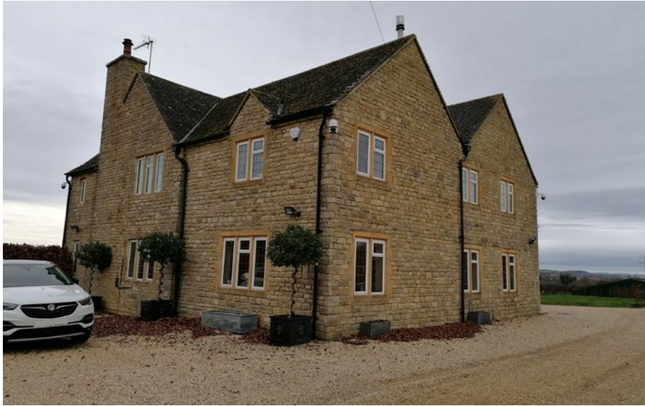
North & East Elevations - As seen from Road.
