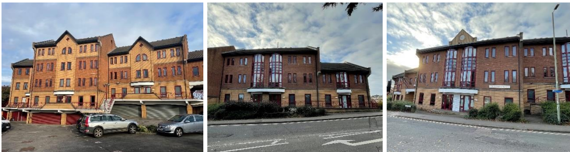
Figure 2: Front and rear elevations of Waterperry Court (bottom row shows with Brethertons signage recently removed)
