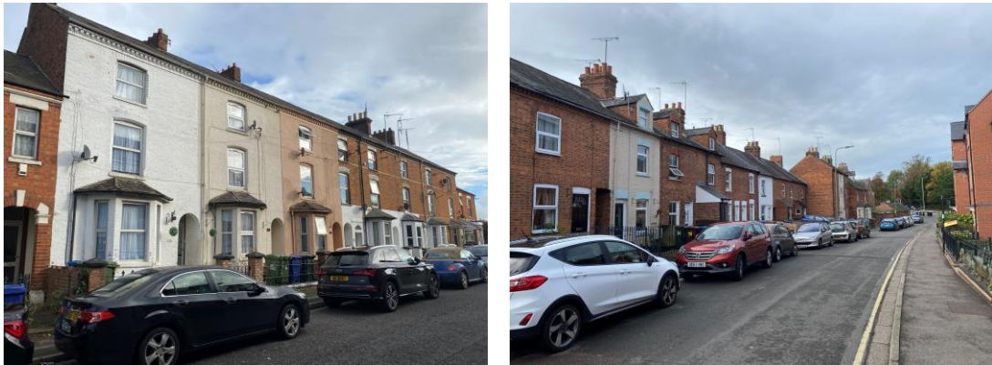
Figures 8 and 9: Characteristic terrace housing within the Grimsbury Conservation Area
