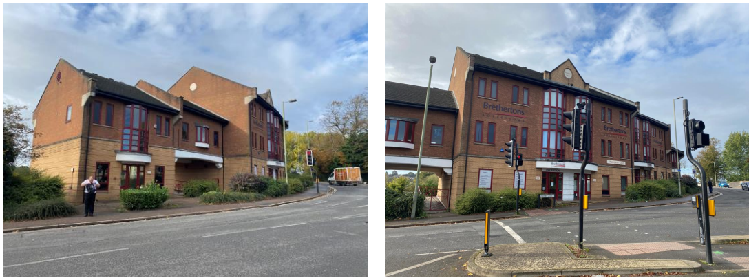
Figures 5 and 6: Existing building present on the site
