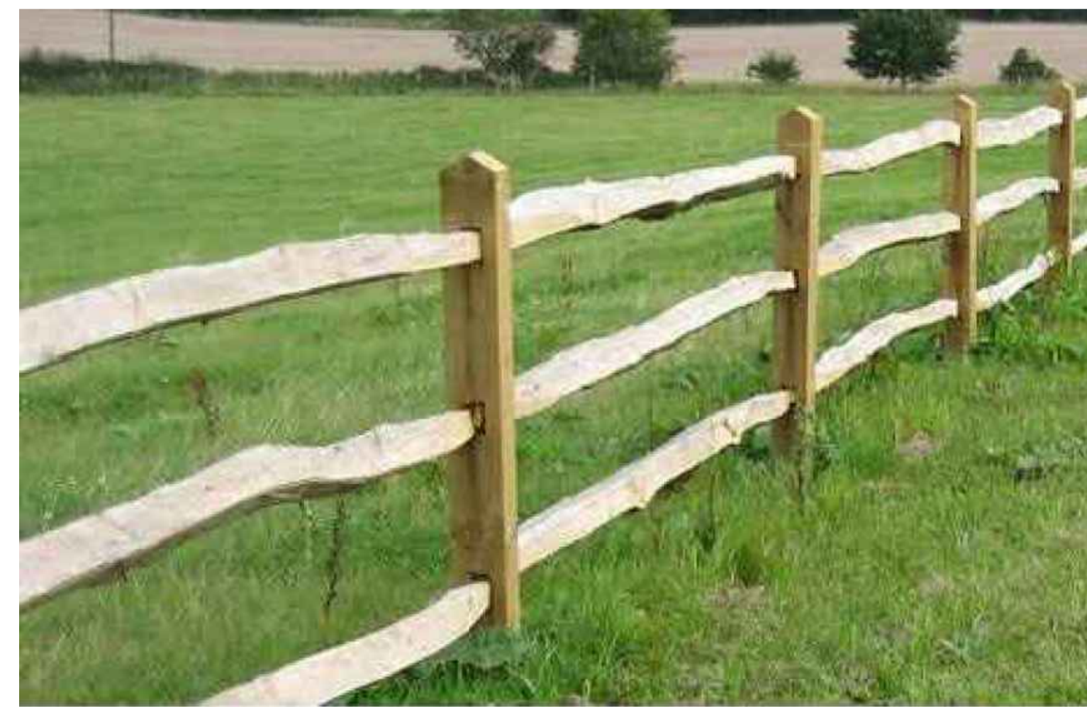
TYPICAL MORTICED TIMBER POST AND RAIL FENCE
