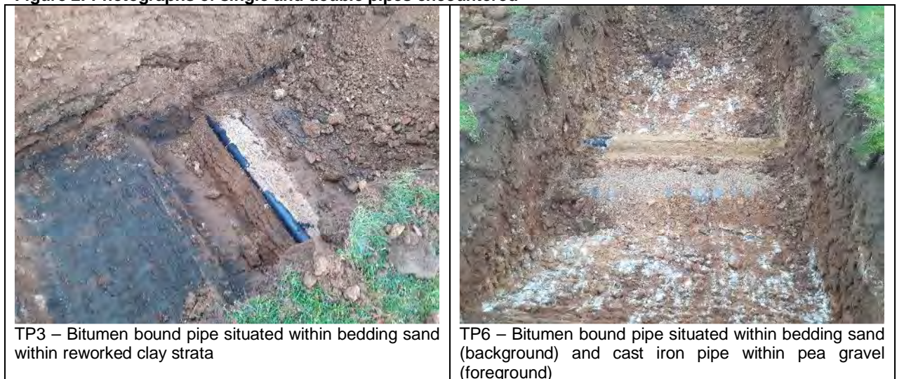
Figure 2: Photographs of single and double pipes encountered
