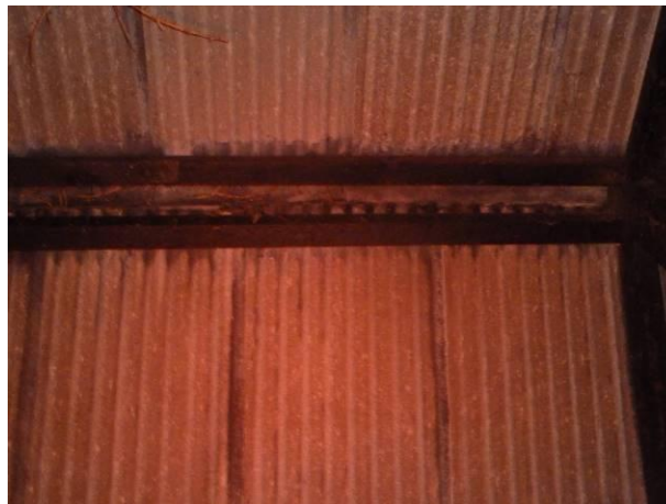
Two central purlins
