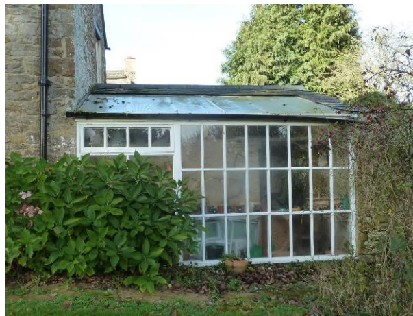
Glazed roof of single storey element
