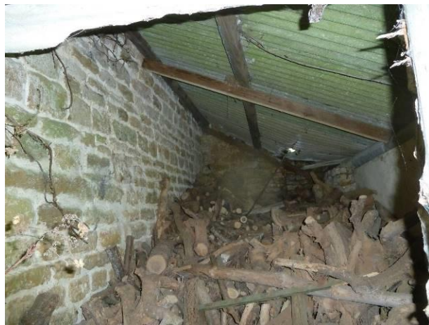
Log store lean to at northern elevation
