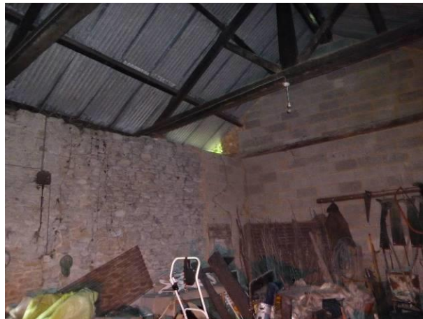
Light ingress at south-east corner
