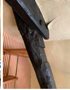
Fig. 18, Detail of truss showing raised collar
