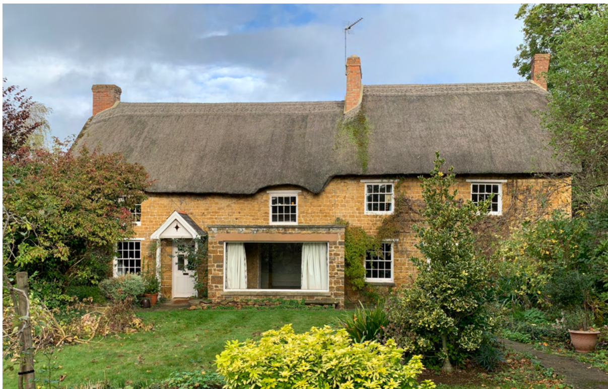
Fig. 1, Ivy Cottage south front
