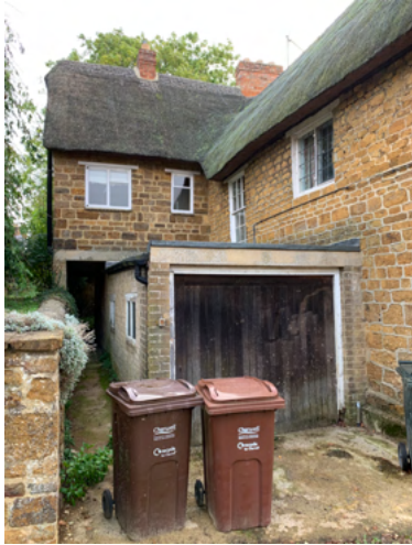
Fig. 3, The modern rear extension.
