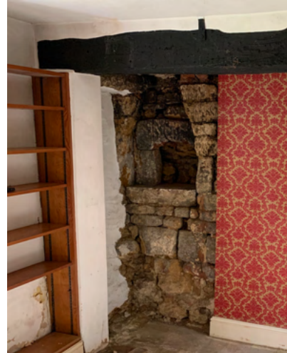
Fig. 5, The interior face of the bread oven with the sitting room fireplace.
