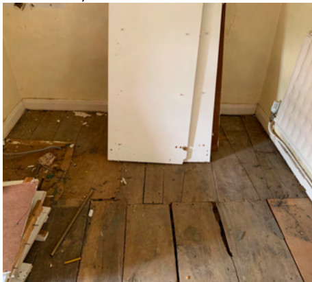
Fig. 19, Bedroom 1 NW corner –boards trimmed and possible early opening covered.
