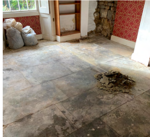
Fig. 9, The newly exposed flagstone floor
