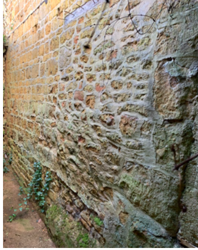
Fig. 4, The chopped and blocked bread oven within the western gable end.
