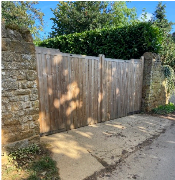
Other similar driveway gates in stone walls to nearby properties within the conservation area
