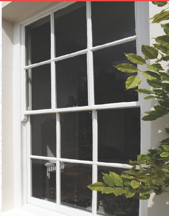
Full treat applied to a vertical sliding Sash
