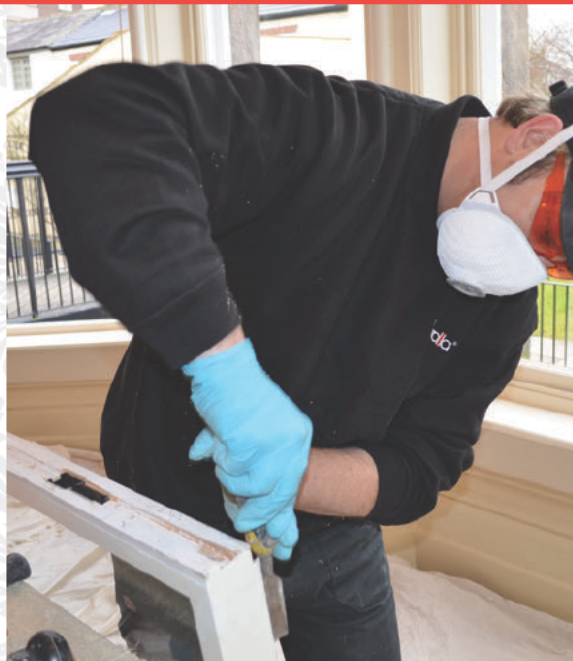
All work is carried out inside with dust sheets.
