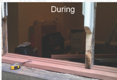
Sill replaced with bespoke new timber and rot cut out from sash frame
