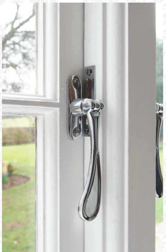
Refurbished Casement window
