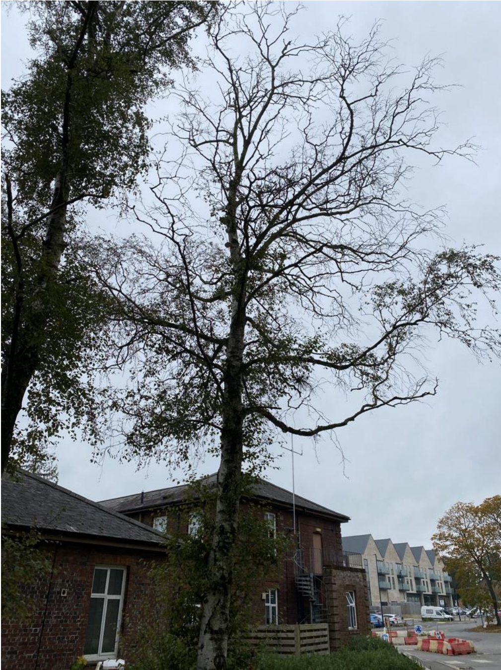
Photo 10: T1 birch. Major deadwood overhanging car park entrance and school footpath.
