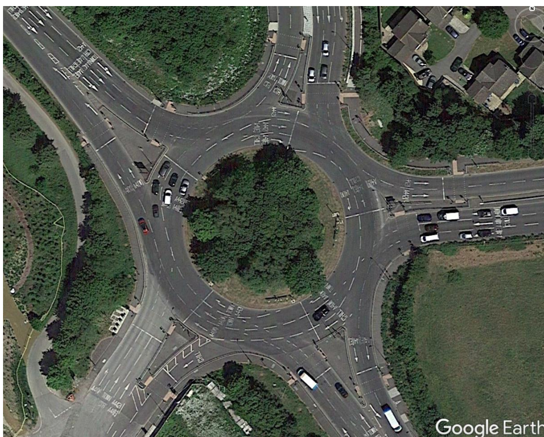
Figure 4.6 A41 / B4100 London Road / A4421 Seelscheid Way / Gravenhill Road Roundabout – Current Layout
