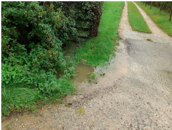
Blocked and hidden drains
