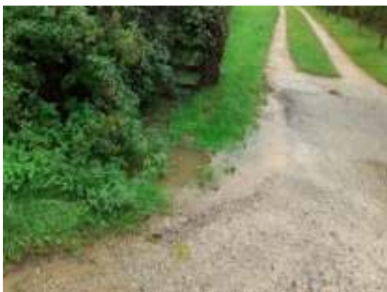
Blocked and hidden drains
