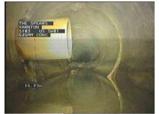
SW01X\_077cb51c-3cbf-4494-be3a-f472d2487bc4\_20220321\_ 094704\_421.jpg, 00:04:46, 15.90 m Connection defective, connecting pipe is intruding at 9 o'clock, diameter: 300mm, intrusion: 35%
