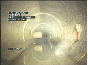
SW01X\_58001230-d6e8-457e-8dd3-c85f2592b01c\_20220321\_ 094555\_583.jpg, 00:03:37, 13.70 m Connection other than junction at 3 o'clock, diameter: 150mm
