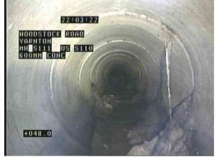
S110Y\_0163fcbb-7220-4892-b9b1-390351d34a93\_20220322\_1 01306\_443.jpg, 00:05:30, 48.00 m Roots, mass at joint, 30% cross-sectional area loss, start
