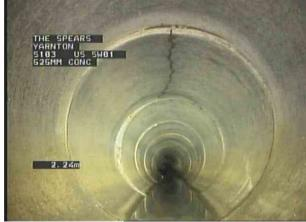
SW01X\_39b2e9aa-0937-4783-ac8b-ef18bf9d43b7\_20220321\_ 094052\_987.jpg, 00:00:39, 2.20 m Fracture, longitudinal at joint at 12 o'clock
