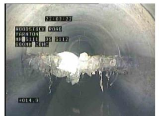
S111Y\_f5efa44c-a95a-4a00-95d4-505e0b2d4aef\_20220322\_1 03249\_221.jpg, 00:01:53, 14.90 m Obstacles, external pipe or cable at 9 o'clock, 100% cross-sectional area loss, Possible service pipe
