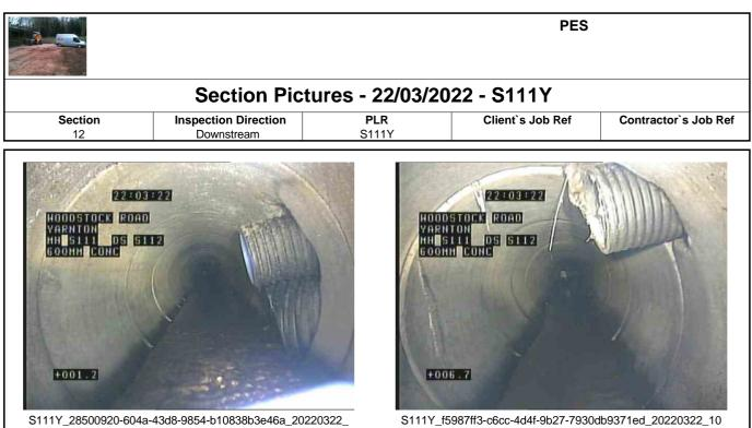
103005\_337.jpg, 00:00:14, 1.20 m Connection defective, connecting pipe is intruding at 4 o'clock, diameter: 150mm, intrusion: 10%
